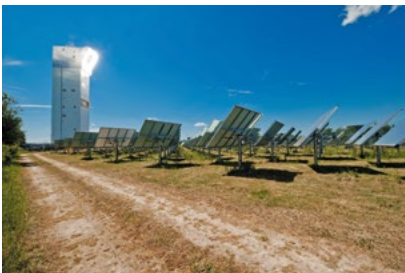
DLR solar tower in Jülich – research power plant for further development of high-temperature process technology
